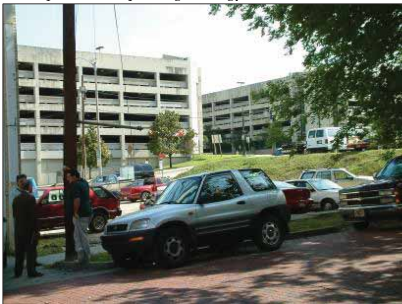
Figure 1.1 – Downtown Baton Rouge Parking Garages
