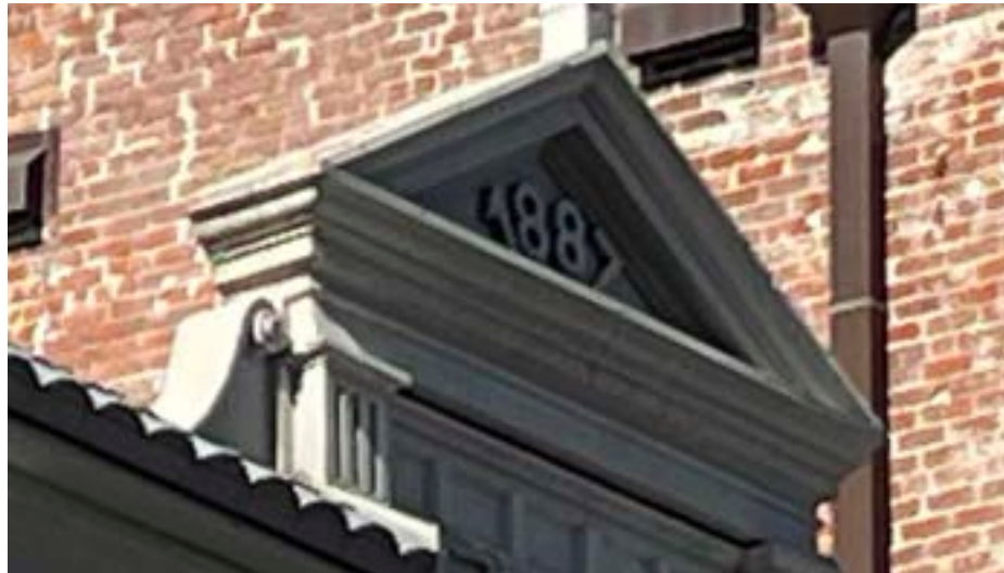
Architectural details can be the subject of a scavenger hunt.
