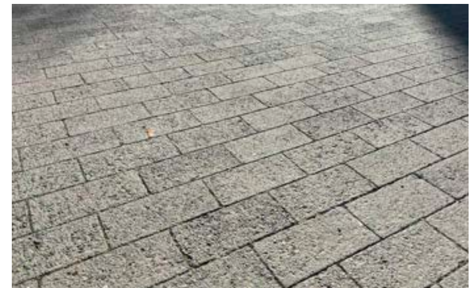
Concrete pavers, Galvez Plaza, east of the Old State Capitol.
